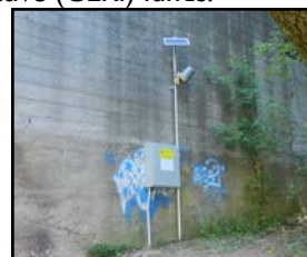
Gage station located just below the Burt Dam
